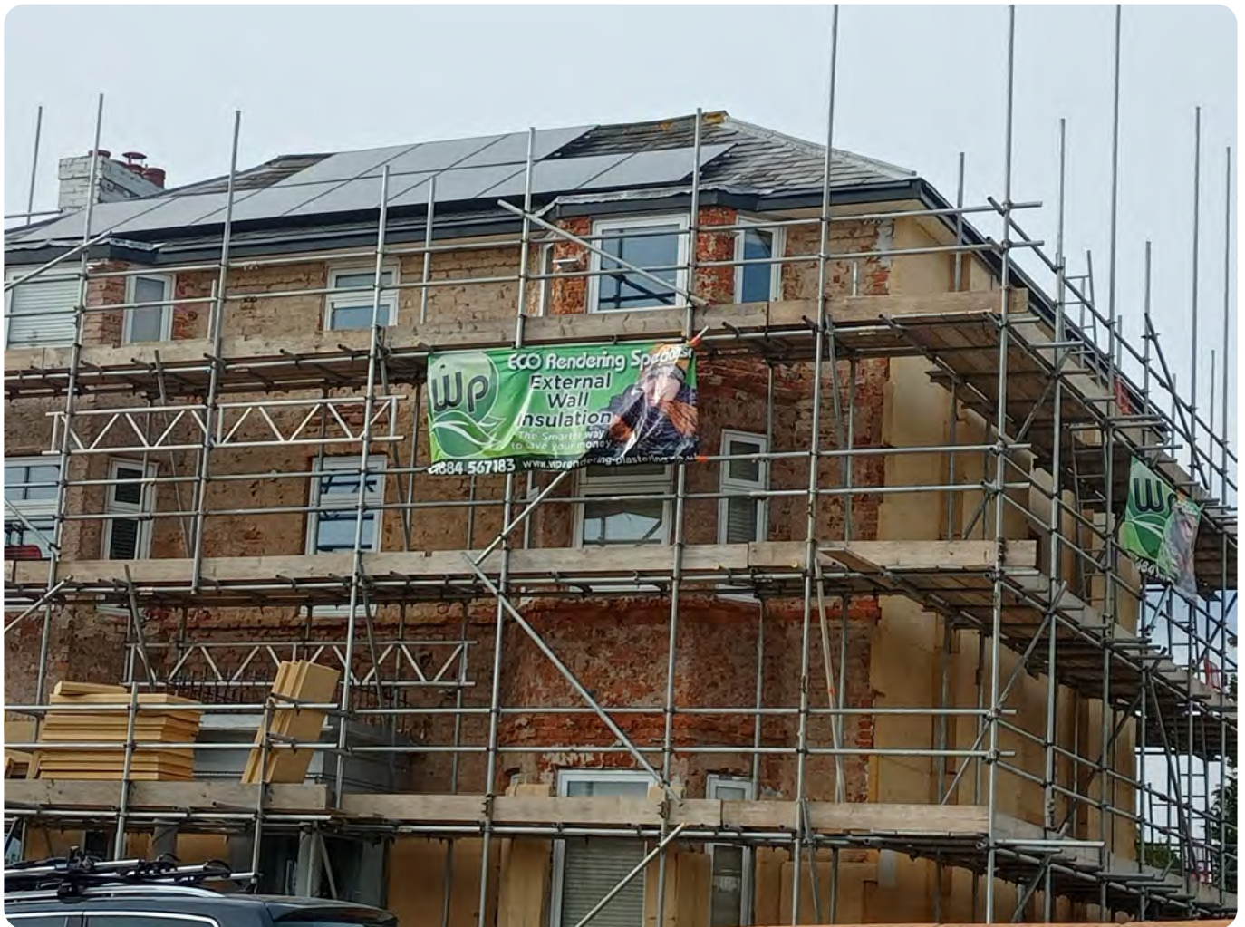
Fitting external insulation and solar panels, West Malvern.
