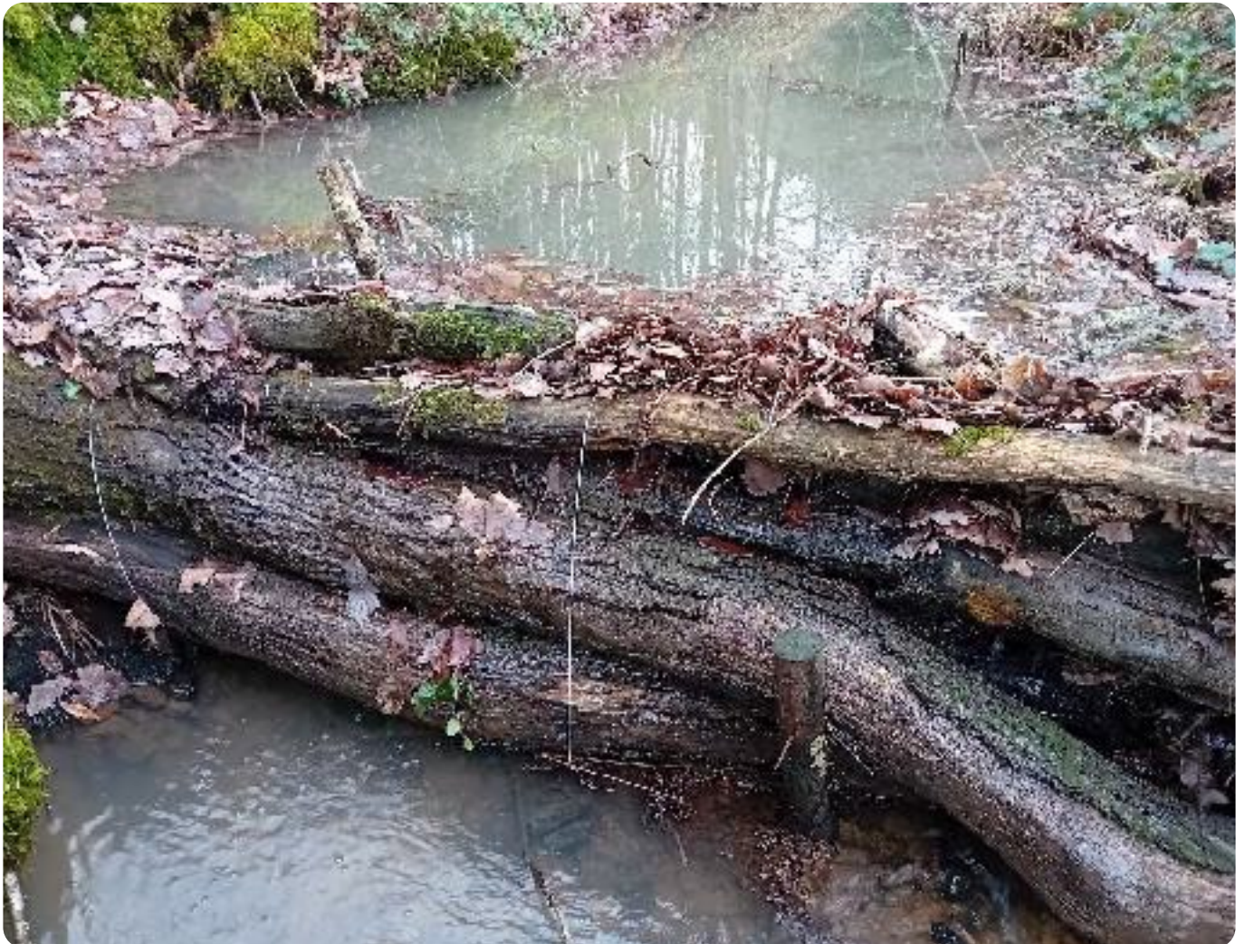
Leaky dam, Worcestershire.
